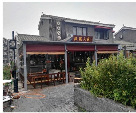
(A2) Nongjiale run by Simatai villagers
