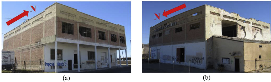
Fig. 1. (a) North-east view and (b) south-west view of the structure [30].
